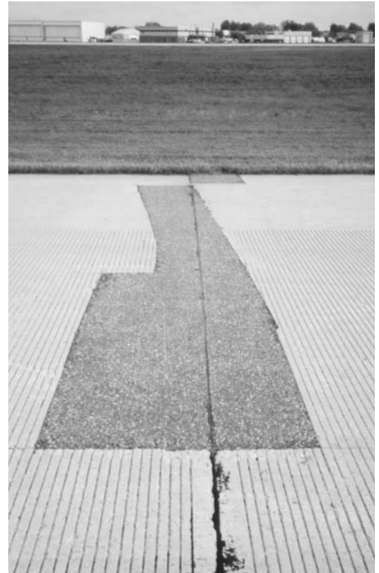
▲ Full depth joint repair. Very good condition.
