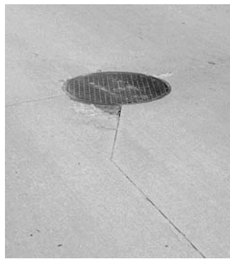
▲ Isolated spall at manhole.
