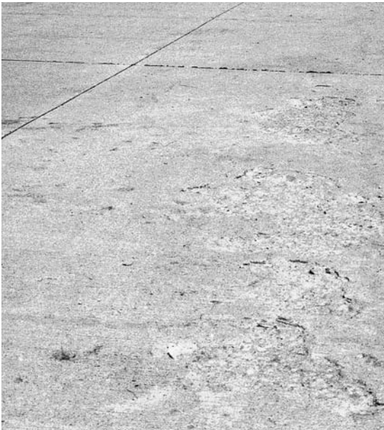
▲ Isolated spall at manhole.
