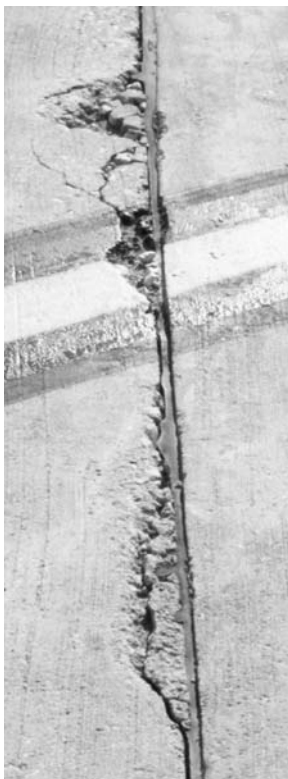
◀ Spalling along a joint.
